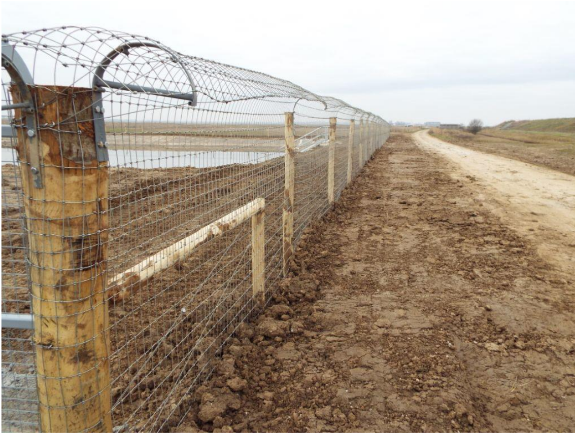
Barrier Fence, RSPB Wallesea
