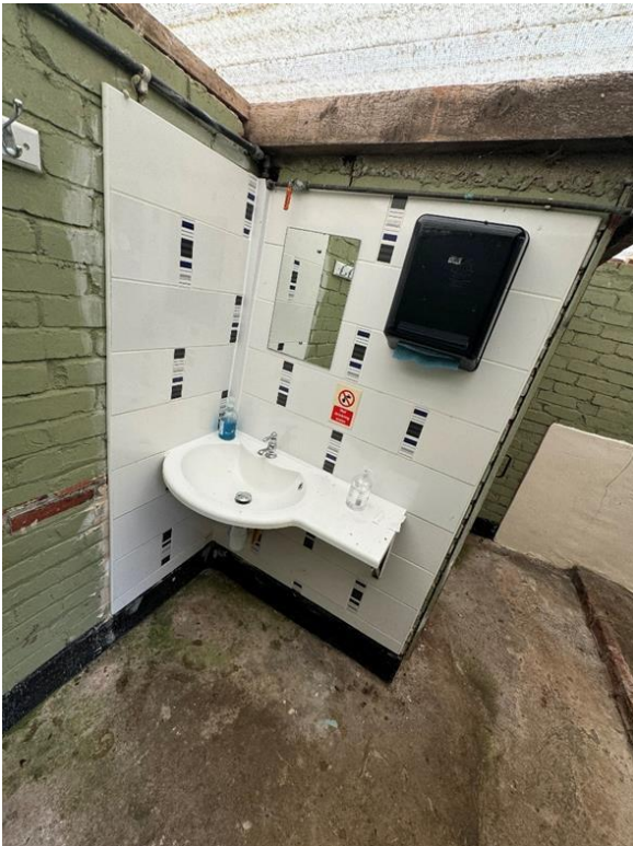
Washing facilities inside toilet block (mens).
